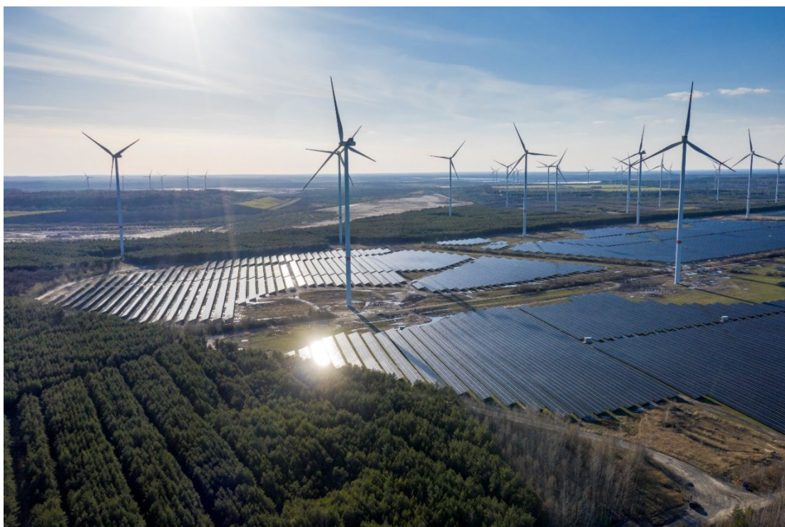
Electricity for households, businesses and for producing green hydrogen: The 300 MW solar park at Lusatia Energy Park in Klettwitz. (Photo: GP JOULE)
