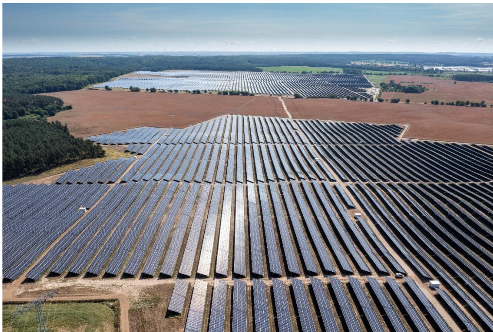
Caption 2: The Boitzenburger Land solar park has a capacity of 180.3 megawatts and will generate approximately 198 gigawatt hours of CO2-free electricity per year on an area of about 170 hectares.
