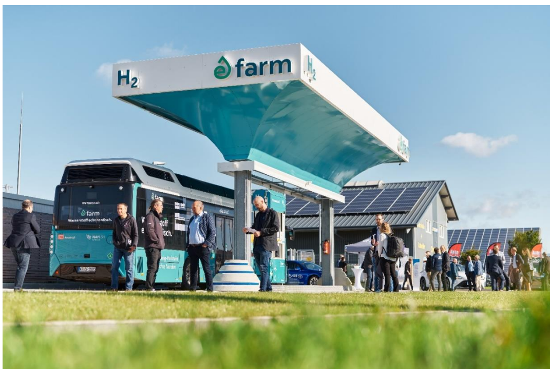
The eFarm hydrogen filling station in Niebüll in Nordfriesland. Photo: GP JOULE
