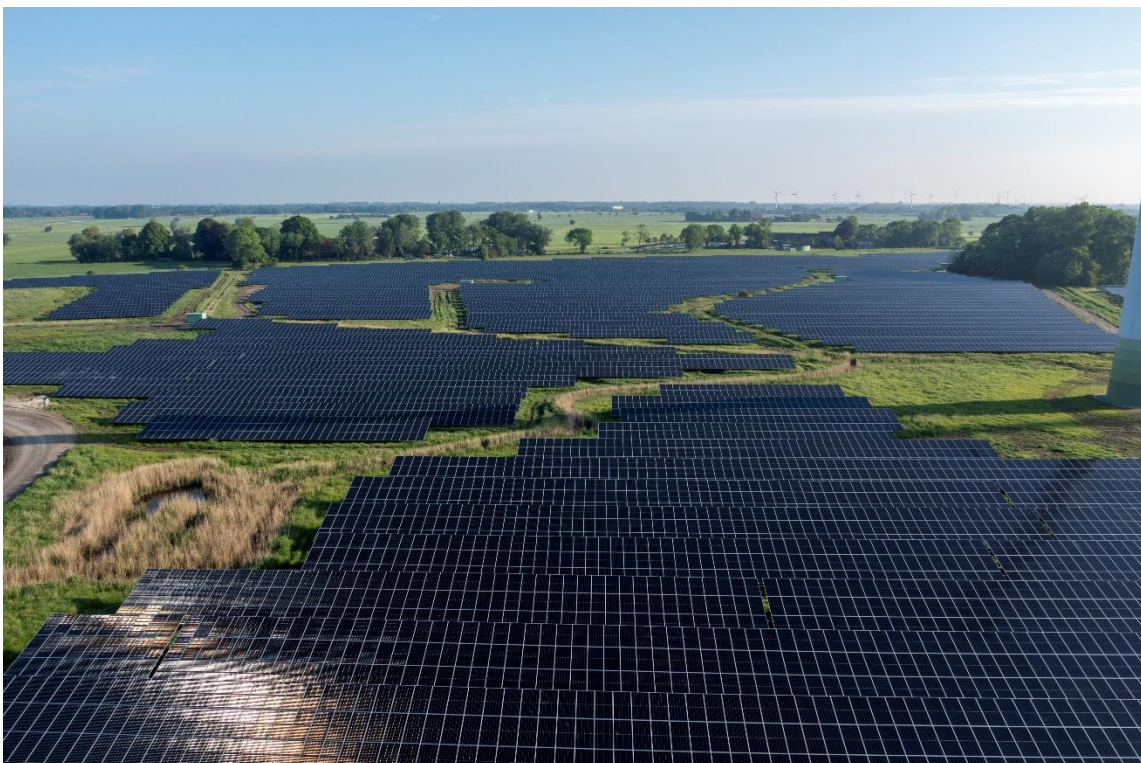
Caption: The Sande solar park is part of the Sande Hybrid Energy Park. GP JOULE's system design enables cost-effective integration into the challenging site.
